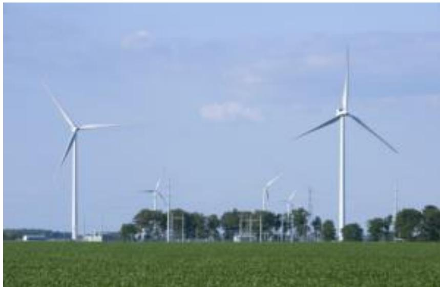
Timber Road Wind Farm in Paulding County, Ohio has 86 wind turbines with an installed capacity of 224 megawatts. That is enough electricity to power approximately 62,000 Ohio homes.
